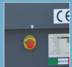
Emergency stop button it shuts down the generating set immediately
